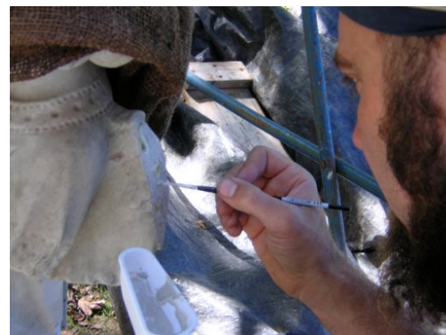
graphs: Repair ready for tion; and, Ap-neat NHL to the process
