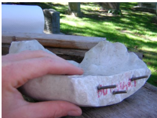
Photo-Two-Step installing repair in
